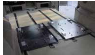
Install OBV Rack base
